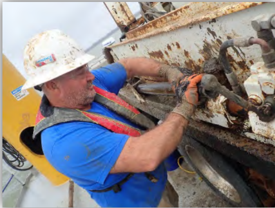
3. Drilling Crew Performed Double Duty (Geotech and Envir Cores) during week.
